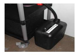
Insert the waste pipe from the sink into the waste water container which can be placed behind or at one end of the unit.
